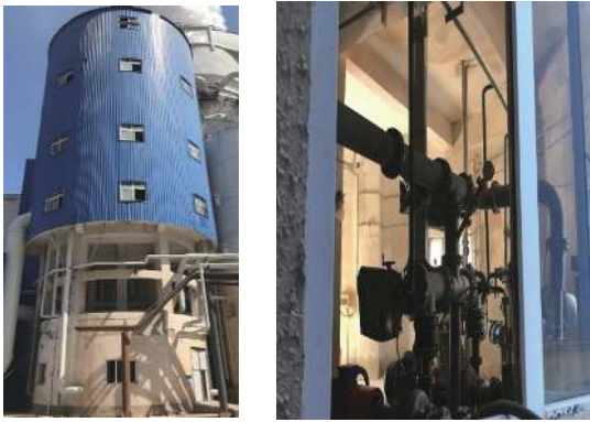
图 1 AFT 结构现场图 Fig.1 AFT structure site drawing
